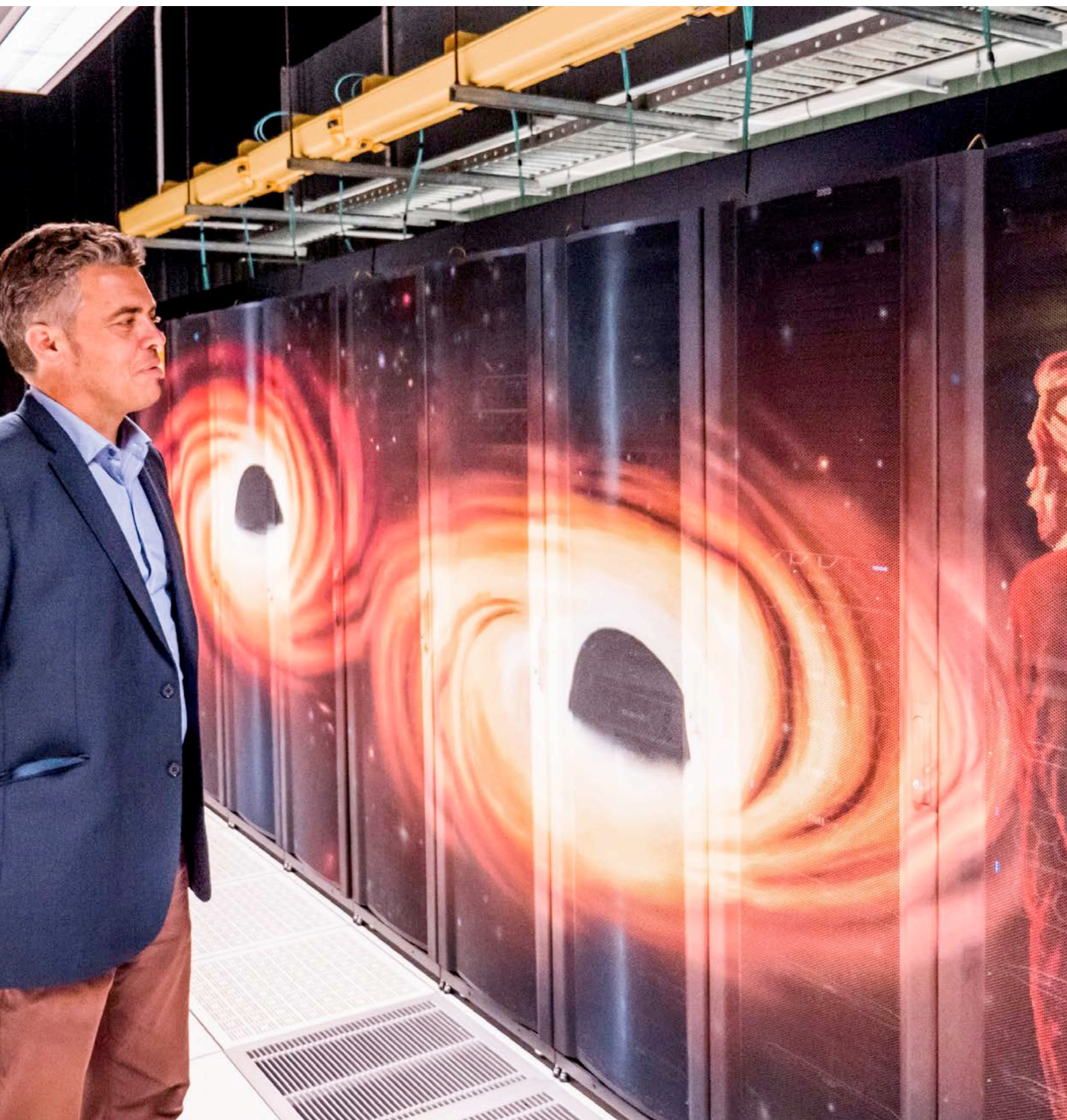
Gravitational Wave Data Centre (GWDC) Program Lead, Jarrod Hurley, with the OzSTAR Supercomputer, located at Swinburne University of Technology. Image credit: Carl Knox, ARC Centre of Excellence for Gravitational Wave Discovery, Swinburne University of Technology.
