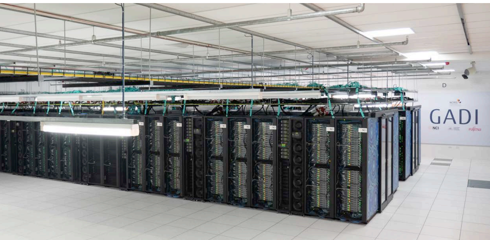
The Gadi supercomputer inside the National Computational Infrastructure data hall. Image credit: National Computational Infrastructure Australia
